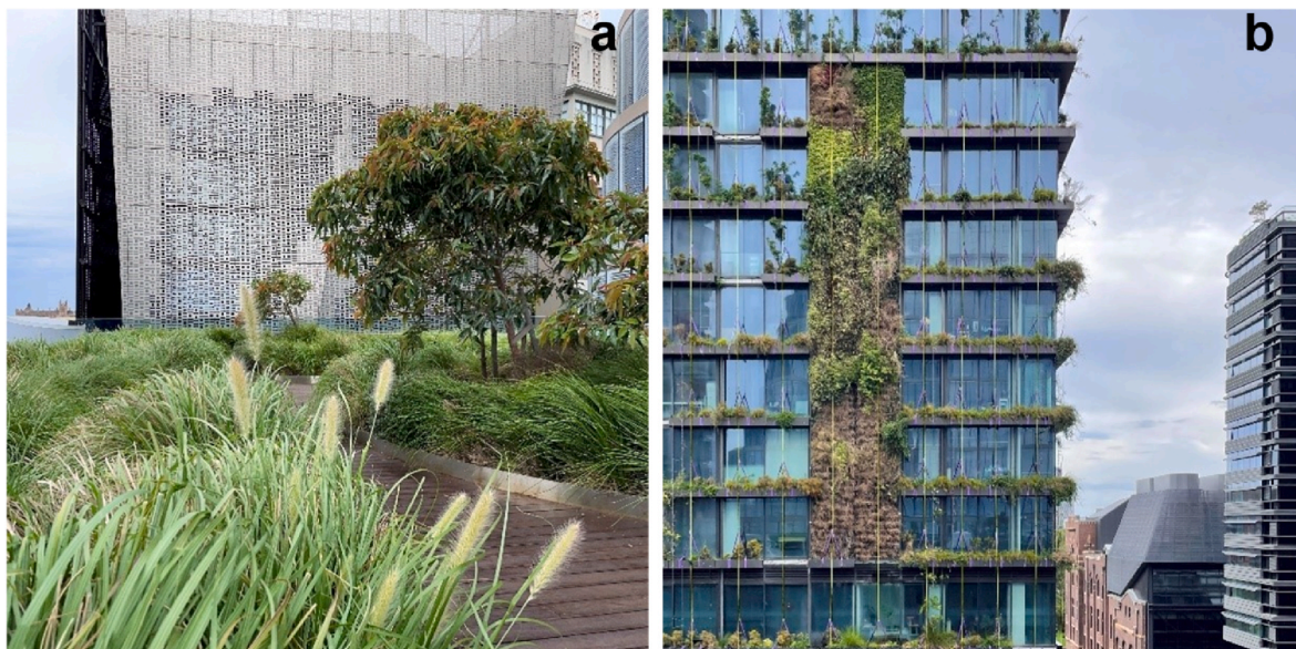
Fig. 3. The UTS Central building with intensive green roofs (a) and the One Central Park apartment building with living green walls (b) in Sydney, Australia. (For interpretation of the references to colour in this figure legend, the reader is referred to the Web version of this article.)
